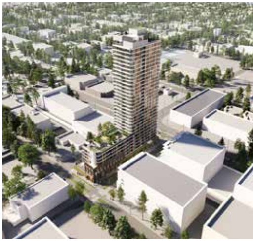
The project. Photo: TransLink
